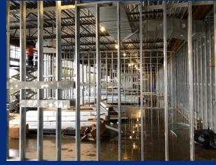
Interior wall framing in progress on 3<sup>rd</sup> level
