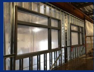
Hollow metal window frames installed overlooking gymnasium
