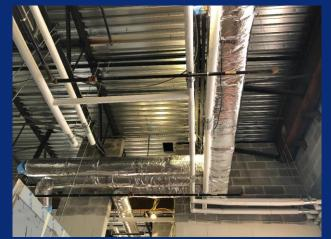
Insulated MEP work ahead of ceiling grid in lower level
