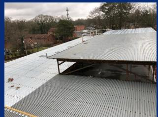
Decking for 2<sup>nd</sup> floor roof and stem lab pop-up installed
