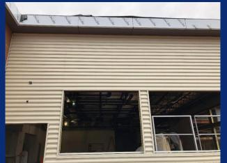
Metal panels, soffits and storefronts installing on south elevation
