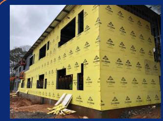
Exterior sheathing on north elevation of main and 2<sup>nd</sup> level east
